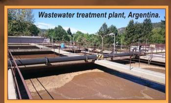
The biological reactors (pictured) continued to function without problems despite receiving 7–12 mm (0.3–0.5 in) of ashfall from the 2015 eruption of Calbuco volcano, 165 km (103 miles) away in Chile. This was partly because the town's storm drains and sewers are well separated, so very little ash entered the plant in raw wastewater. Photo by Daniel Blake.
