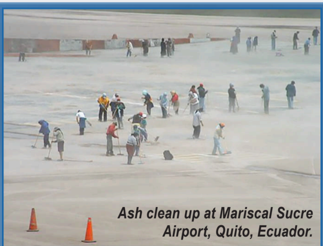
It took 500 people at least 7 days to clear ash from the airfield using brooms when 4 mm (0.2 in) ash accumulated following the 2002 eruption of Reventador volcano. Photo by Mariscal Sucre Airport, Ecuador.
